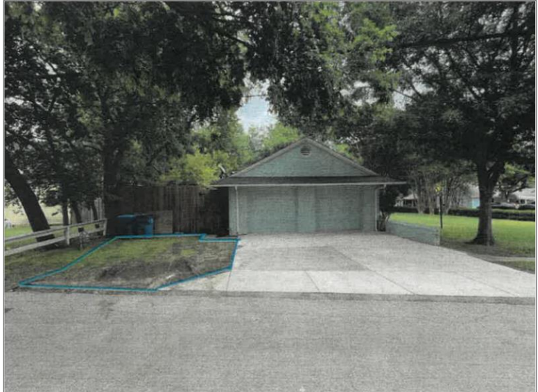
PICTURED ABOVE: CONCRETE DRIVEWAY EXPANSION ALONG N. FANNIN STREET SHOWN IN BLUE
