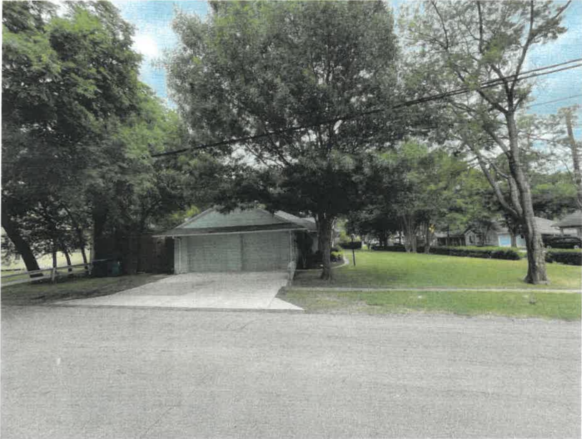
Picture 3: Driveway and yard view of 303 Williams off Fannin St.
